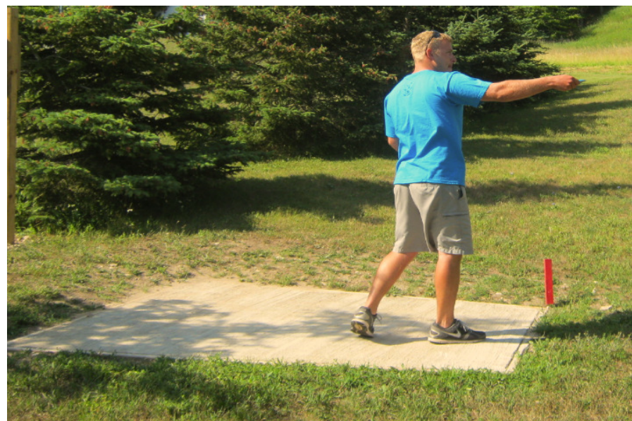
EXAMPLE CONCRETE TEE PAD AT MT. MCSAUBA DISC GOLF COURSE IN CHARLEVOIX
